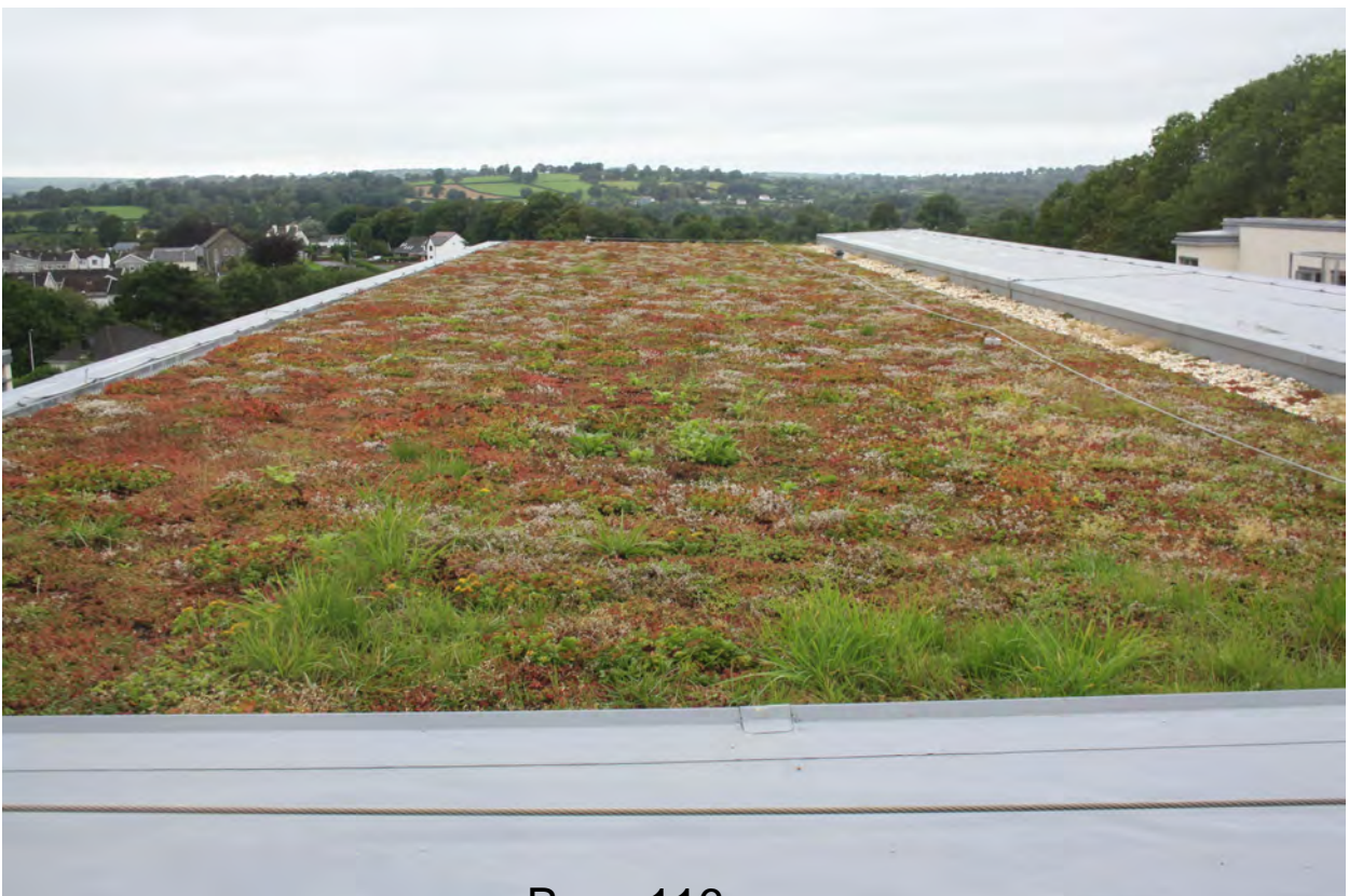
Picture 5.4 Living Roof (Copyright Chris Jones)
